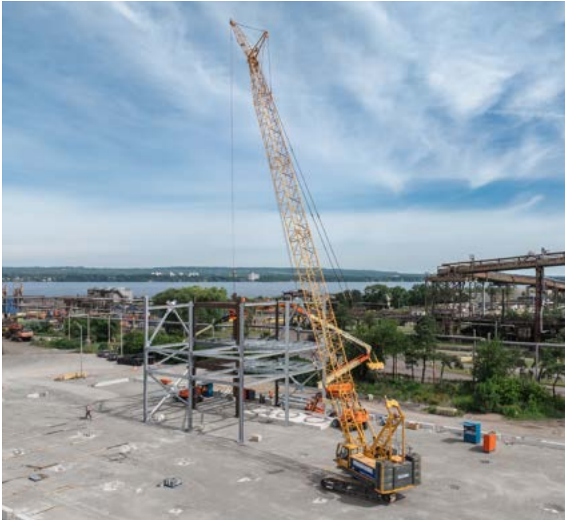
Building new sugar processing plant at Pier 15, HOPA Ports
