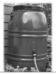
Rain barrels typically include a leaf & mosquito filter, spigot, and overflow hose.
